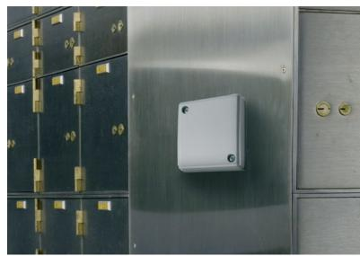
Another example of bank security involves interlocking. When a staff member unlocks a vault, the door to the secured area simultaneously locks. This prevents anyone else from gaining entry until the vault is once again locked. This ensures the safety of staff members and the security of vault contents.
